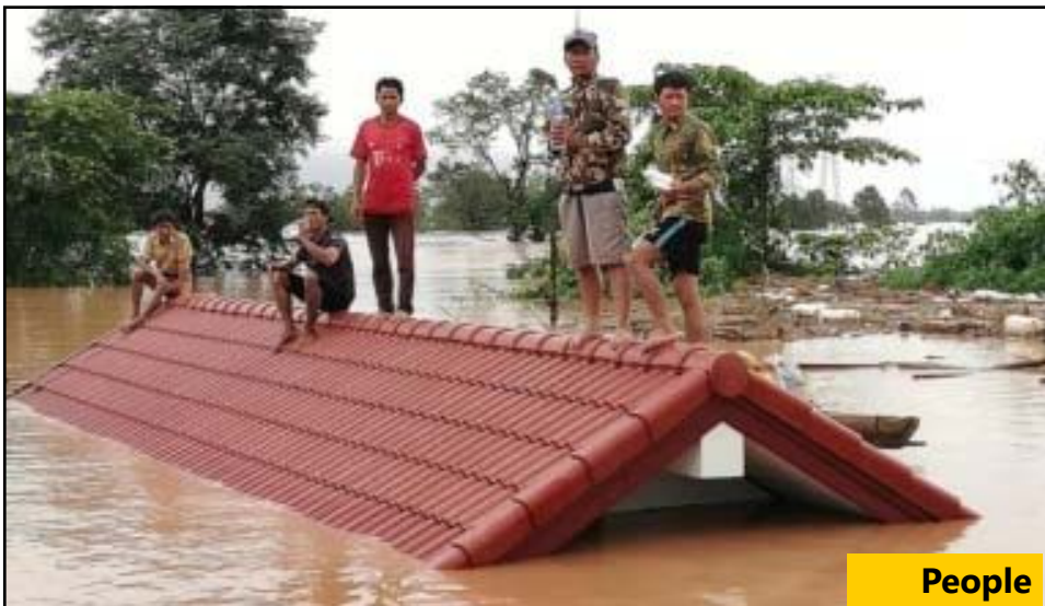
Failed Laos Dam
